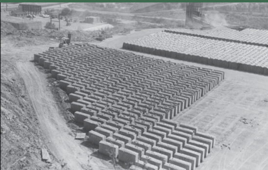
Monterey Park Plant 1950
