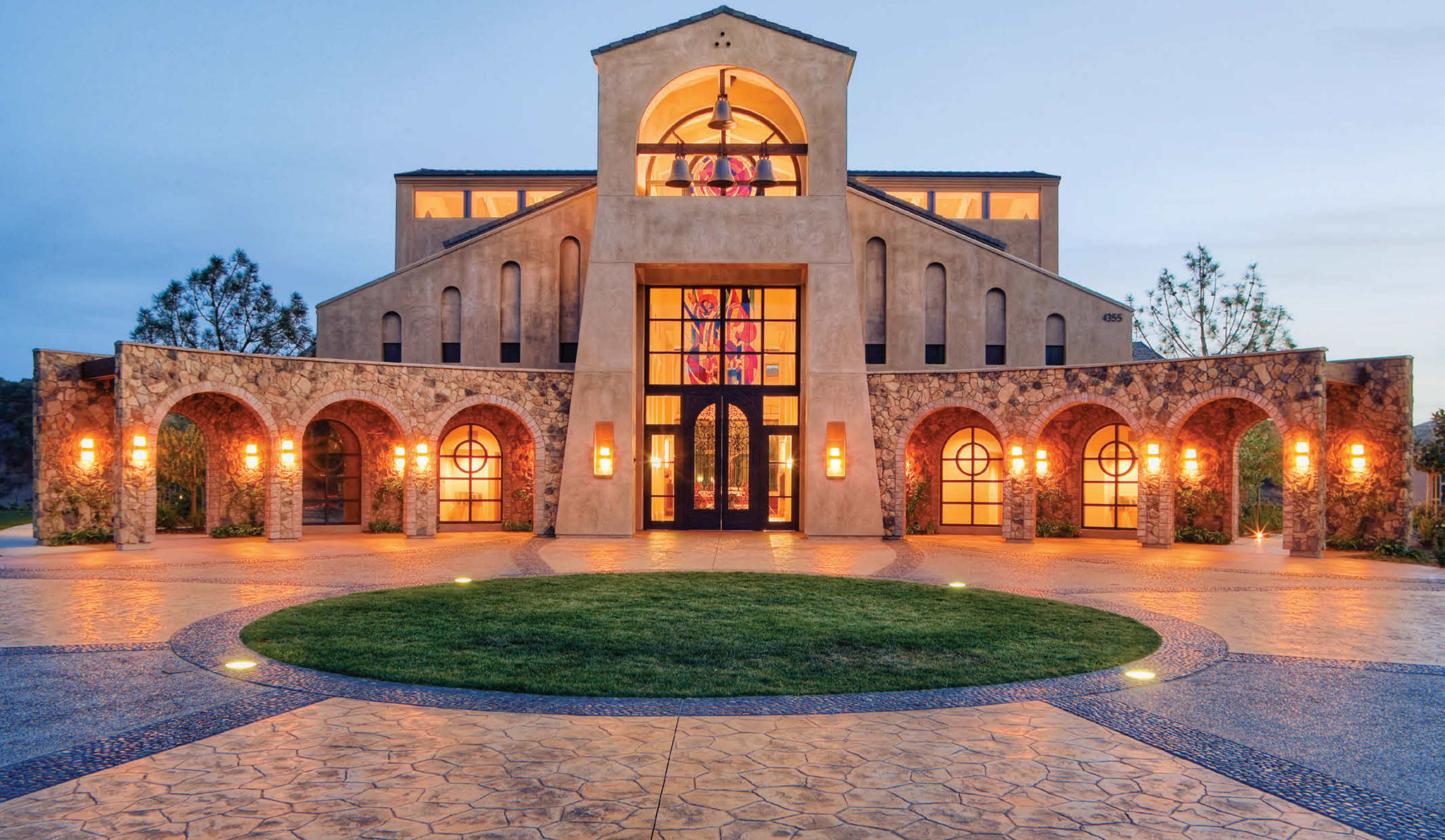
Cognac Country Rubble (pg. 48) with an overgrout technique.
