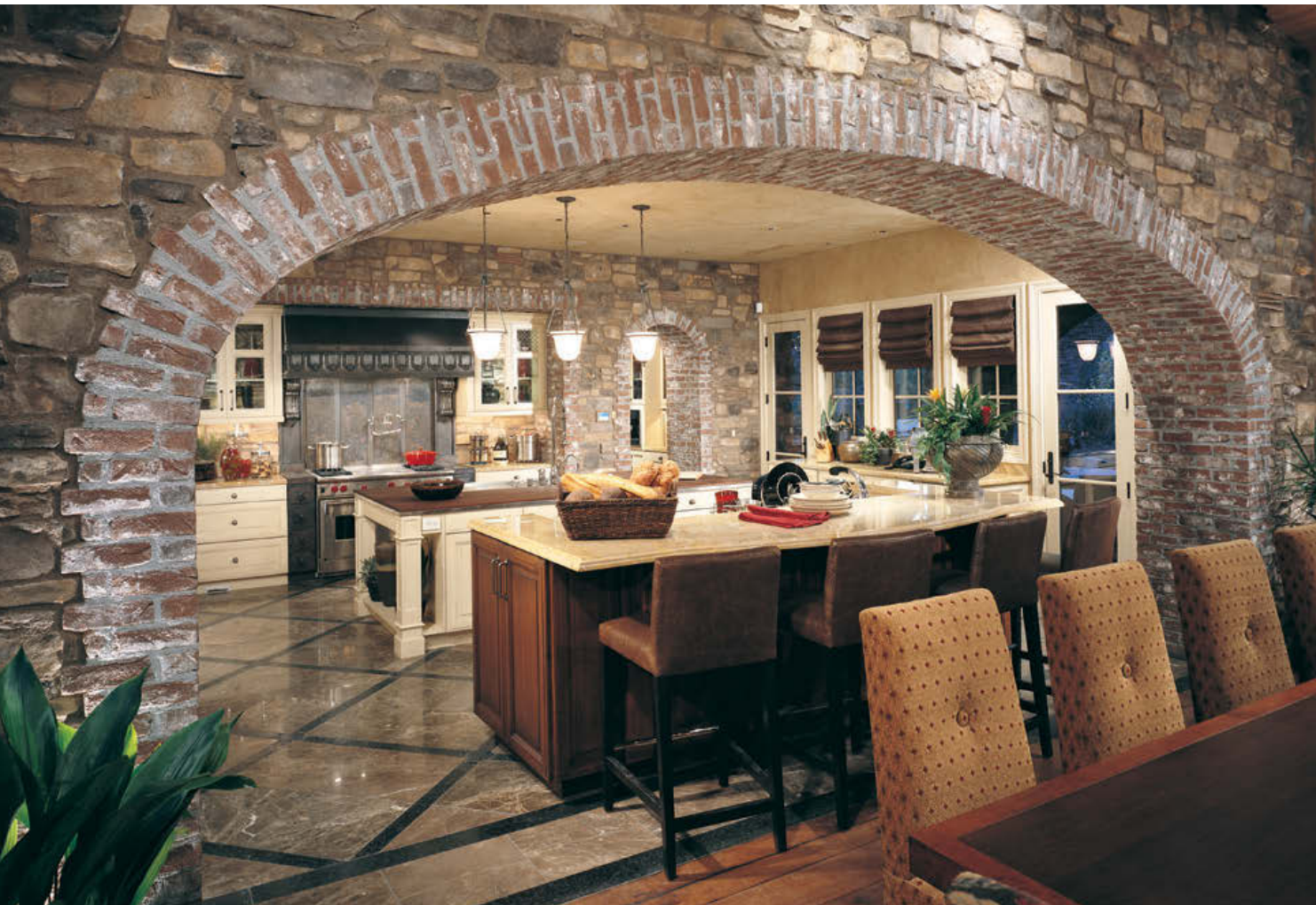
Santa Maria Cypress Ridge (pg. 48) with an overgrout technique.
