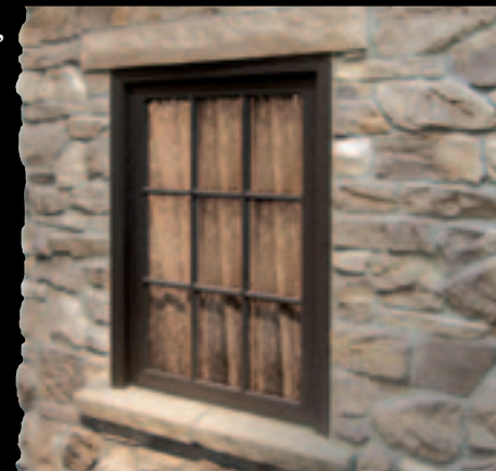
Split Stone Sill - Volterra (Below Window)
